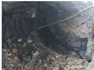
Existing Manhole Example
