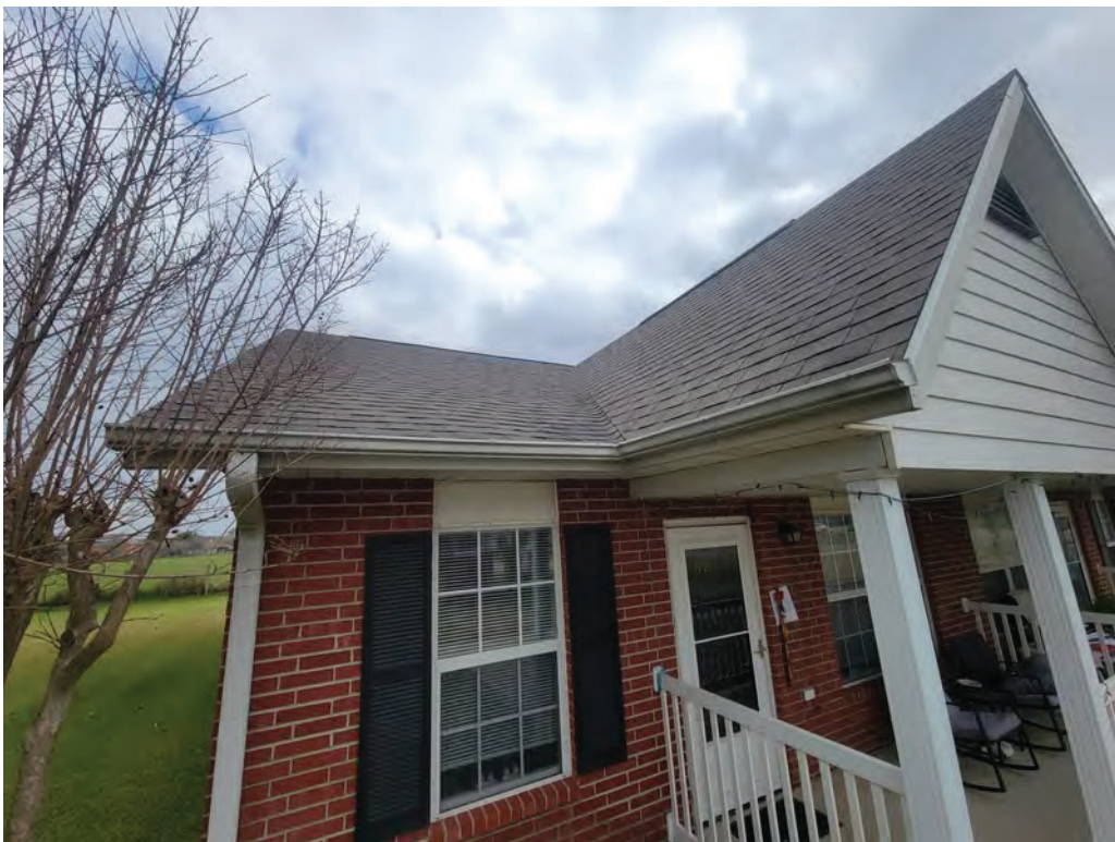
10. Asphalt shingle roofing
