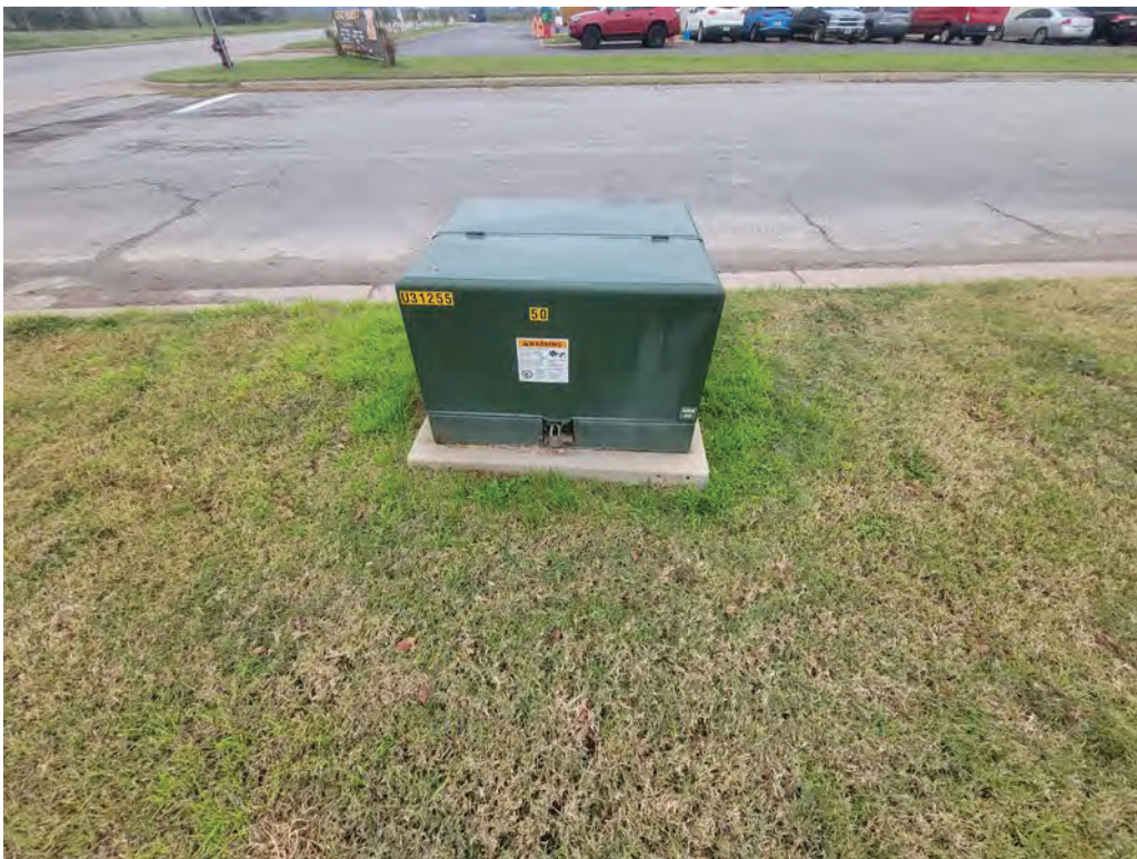
84. Pad-mounted transformer
