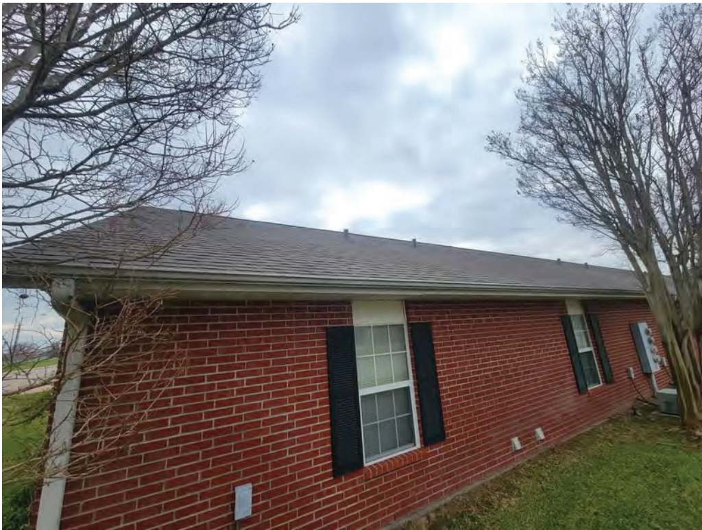
9. Asphalt shingle roofing
