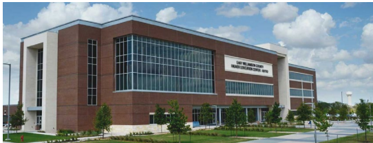
TSTC Campus in East Williamson
