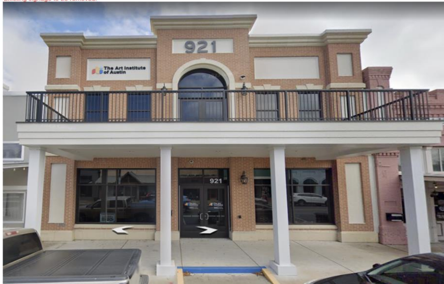
Existing signage to be removed.
