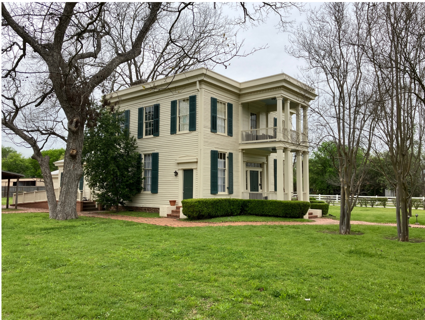
Crocheron House; View looking Northwest from Wilson Street at the front and side elevation Photo 2023 GFA
