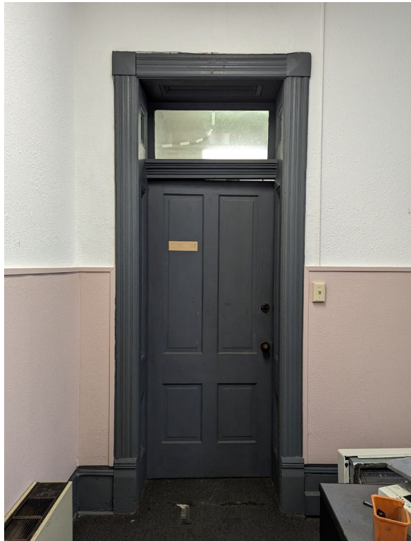
Photo 11: Interior door assemblies and finishes will be restored.
