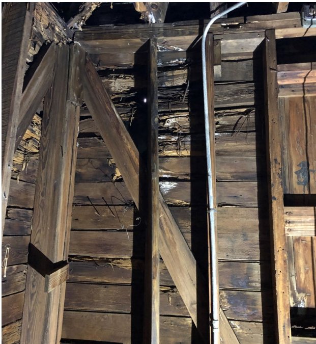
Photo 5: Existing conditions at tower framing
