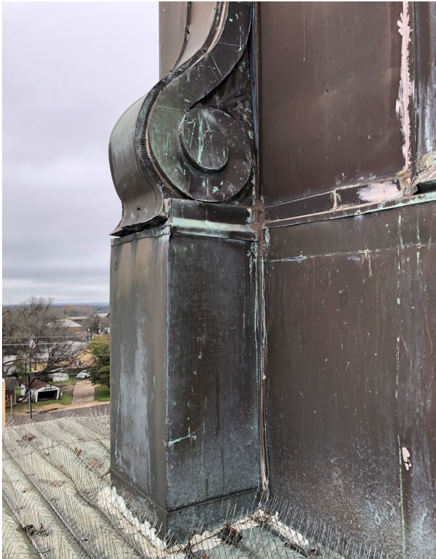
Photo 3: Detail of existing sheet metal cladding
