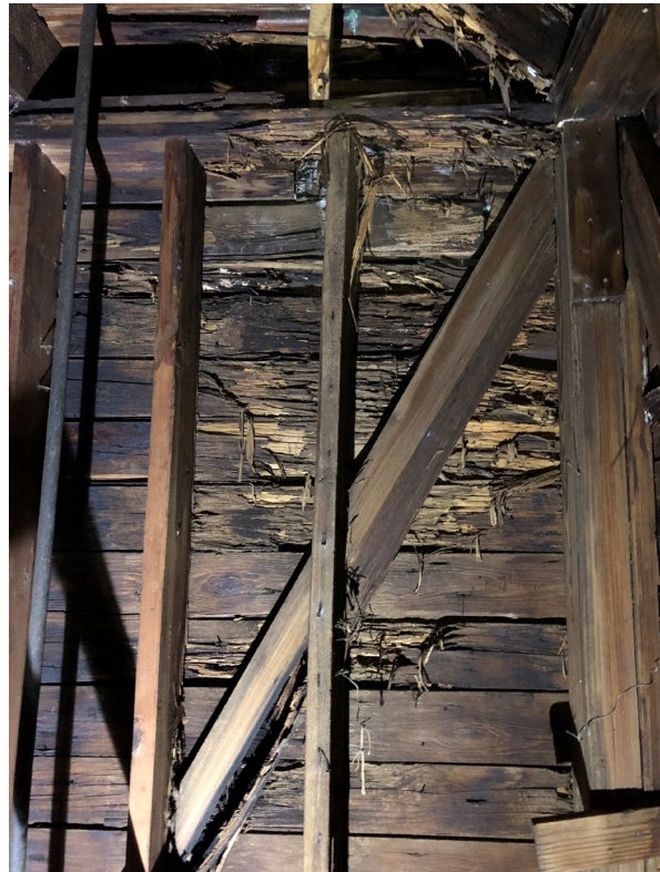
Photo 4: Existing conditions at tower framing
