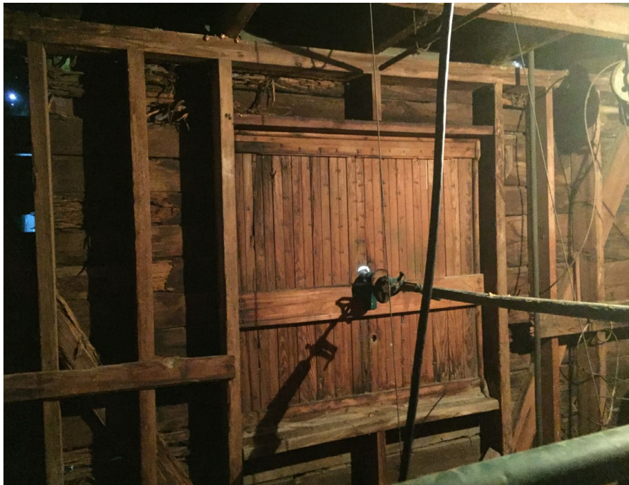
Photo 7: View of clockworks and interior wood framing
