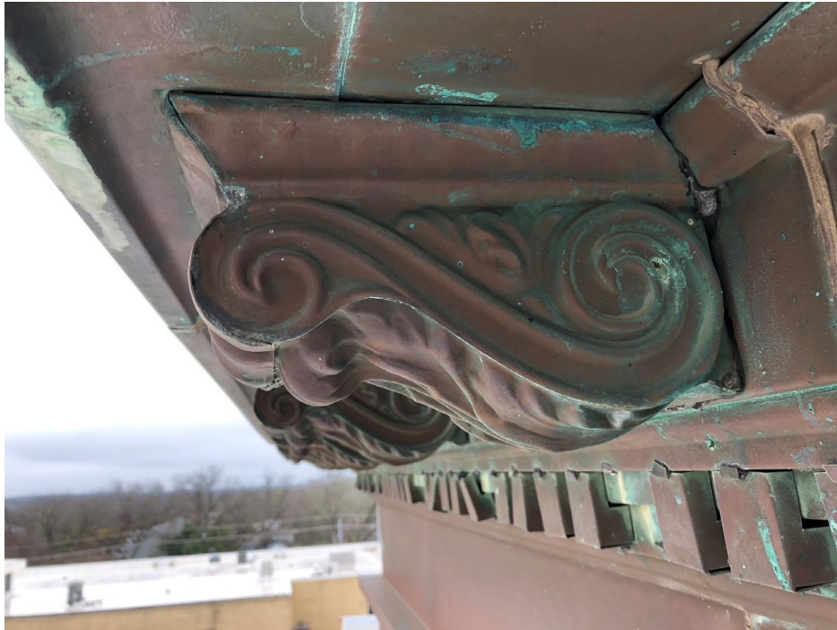
Photo 6: Detail of existing sheet metal cladding
