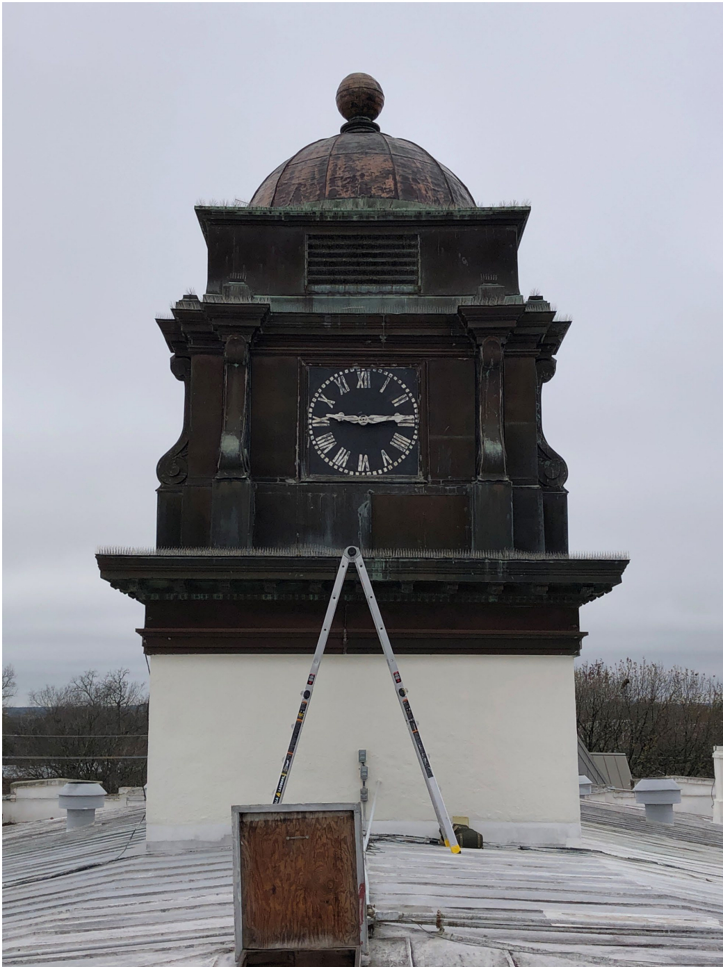
Photo 1: Courthouse tower, existing conditions
