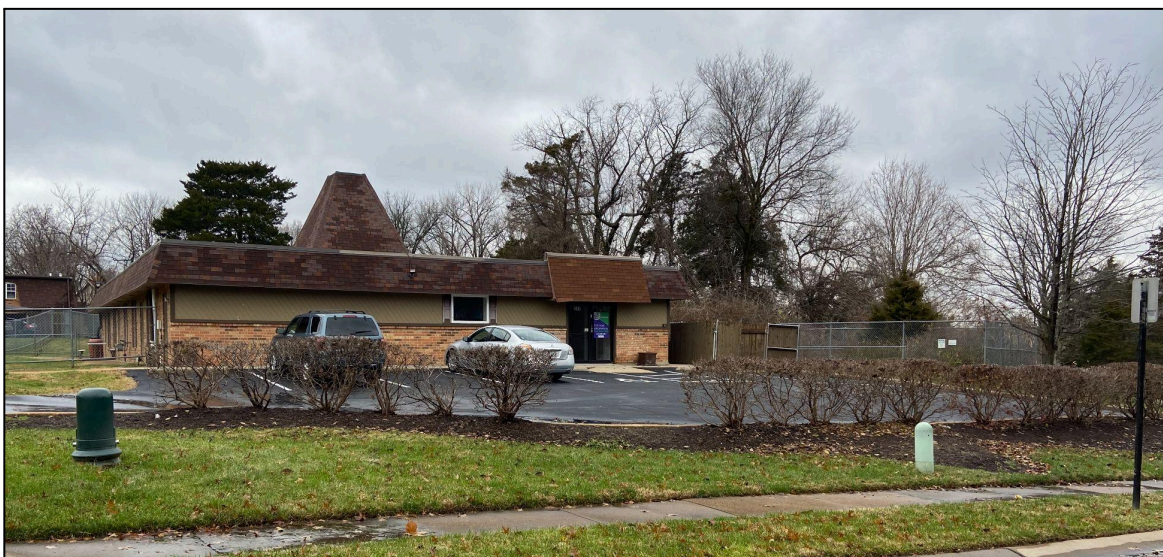
Figure 2 - Street view of the development
