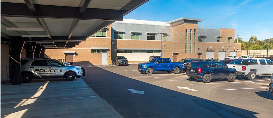
City of Creve Coeur New Police Station, Parking Canopy
