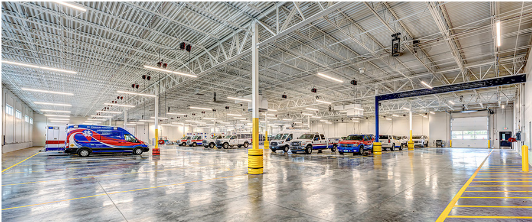
St. Charles County Ambulance District, New Headquarters & Operations Center
