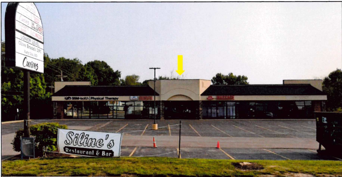
Figure 2 – Street view of the development. The restaurant would be located in the center of the development, as indicated by the arrow.
