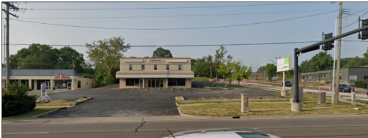
Figure 2 - Street view of the development
