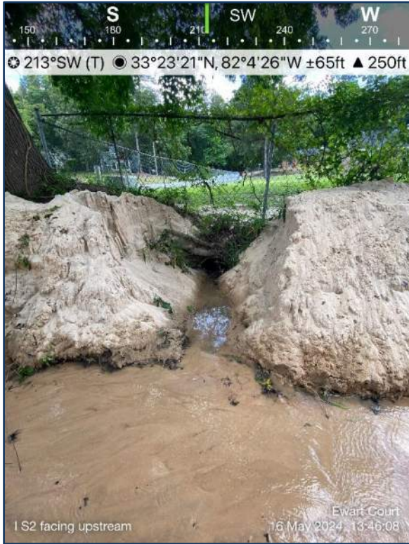
Photograph 5: Embedded culvert outfall structure at upstream reach adjacent to Woodlake Road.
