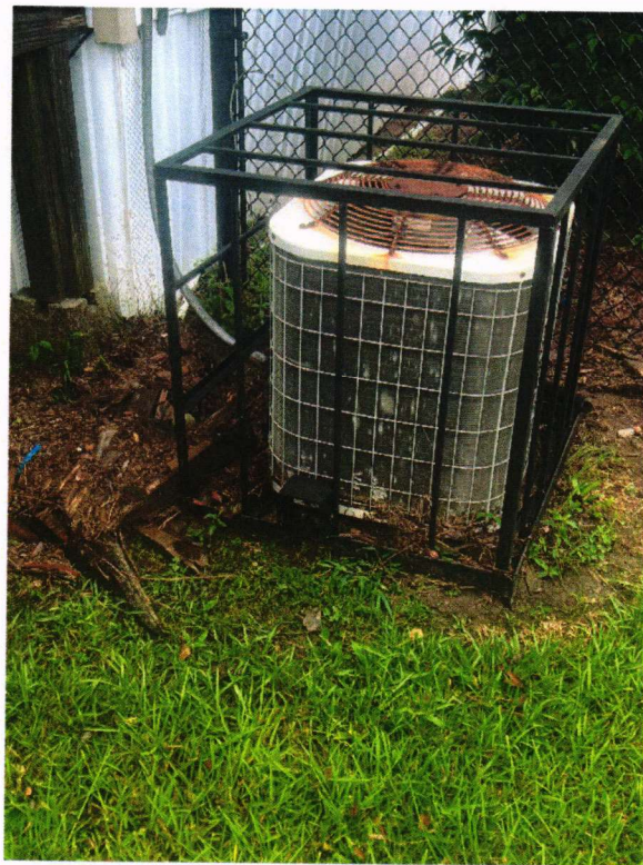
Photo 14. Evidence that HVAC has been submerged.
