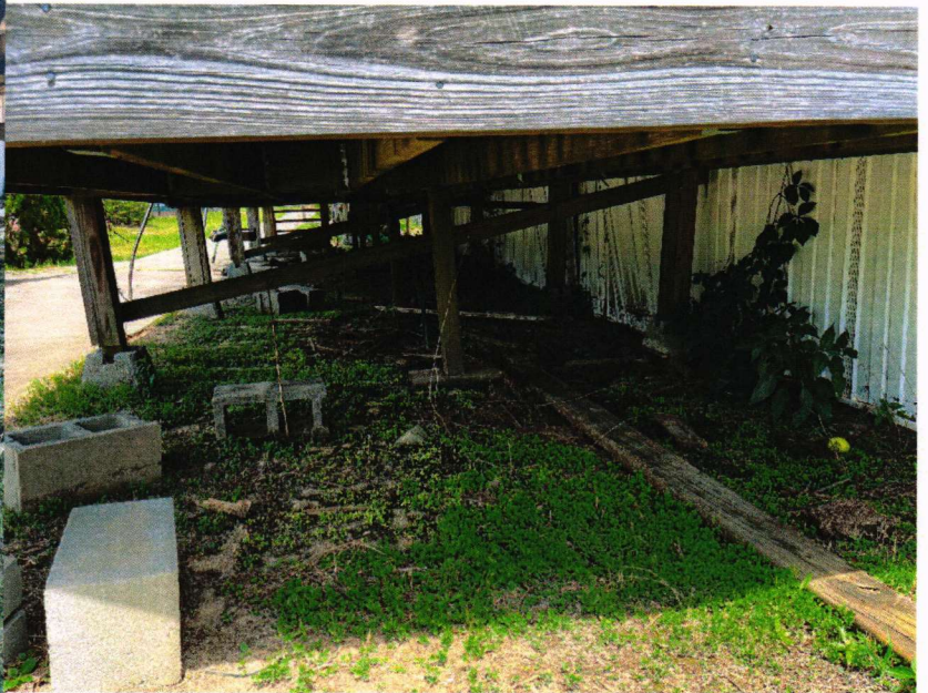
Photos 6, 7, 8, and 9. Unstable support columns.
