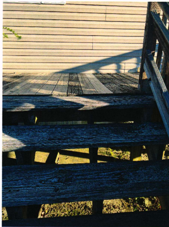
Photo 2. Front stairs and trip hazard.
