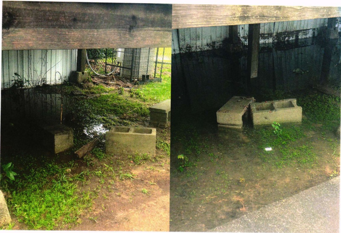
Photos 12 and 13. Standing water under decks.
