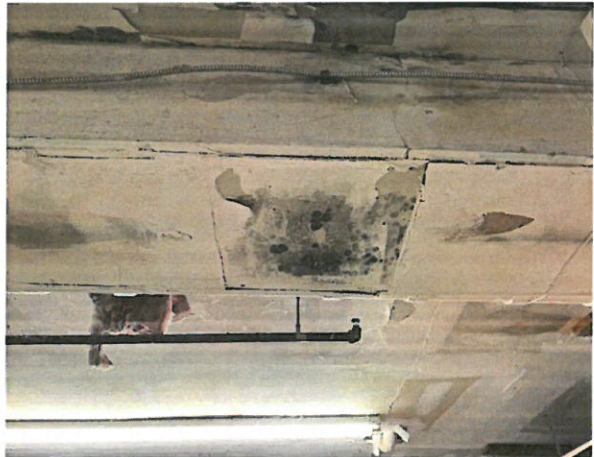
4, Staining Indicative of Mold Colonization Drywall Ceiling
