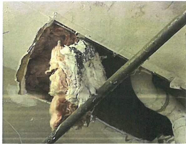
2, Staining Indicative of Mold Colonization on Insulation
