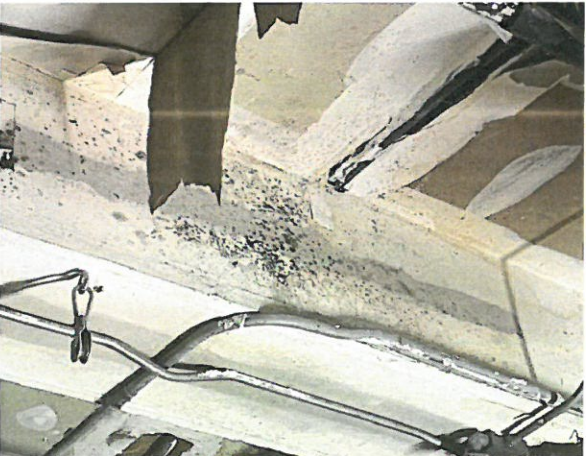
5, Staining Indicative of Mold Colonization on Ceiling Beam
