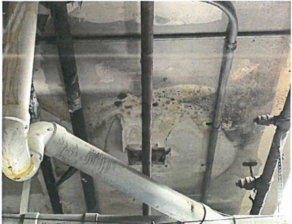
6, Staining Indicative of Mold Colonization Drywall Ceiling
