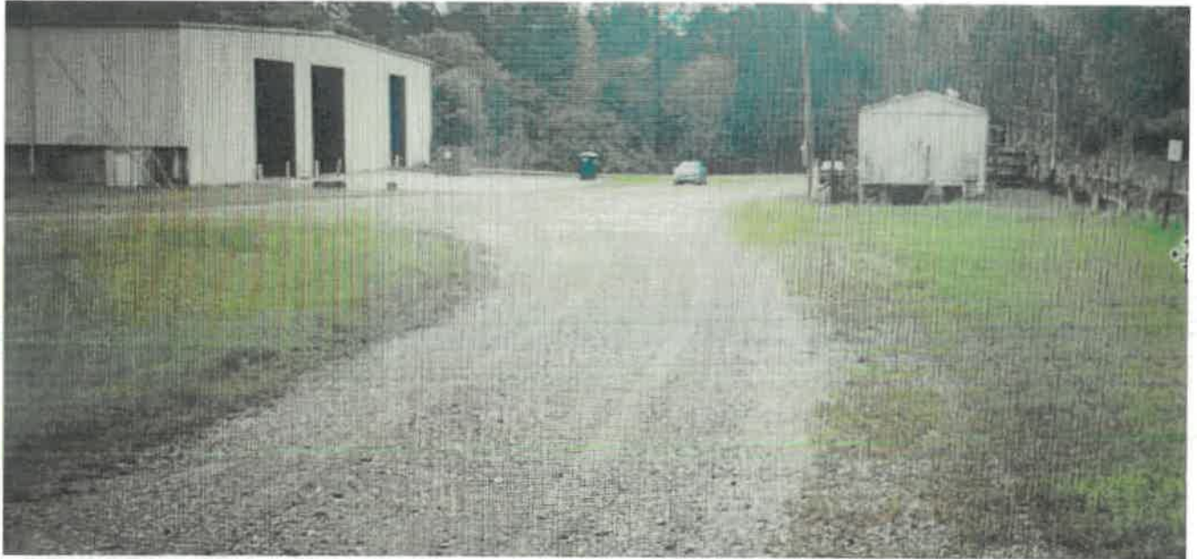
Photo 1: Entrance to Facility at 3946 Goshen Industrial Blvd.
