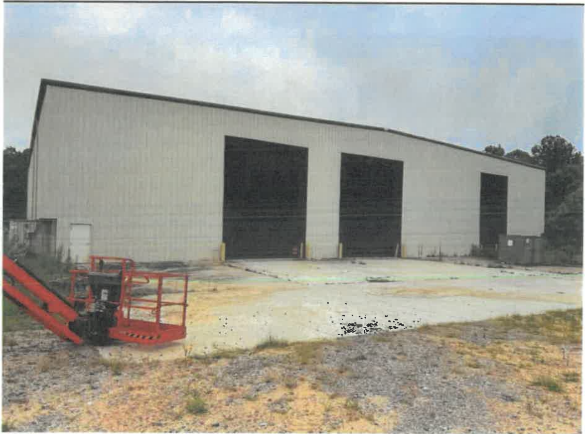
Photo 2: Front of existing Transfer Station Building
