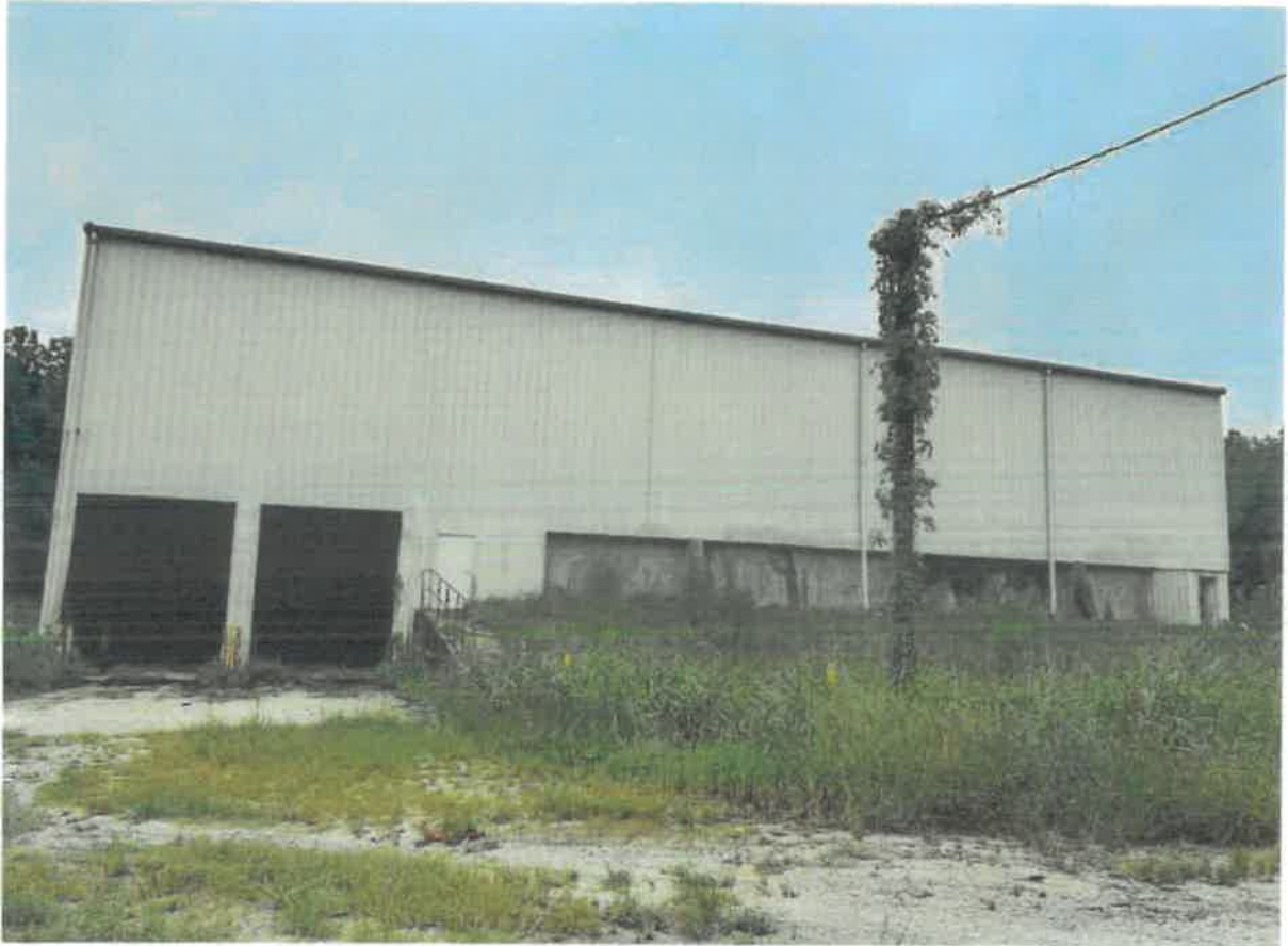
Photo 3: Side of existing Transfer Station Building, including Truck Pit Entrances.
