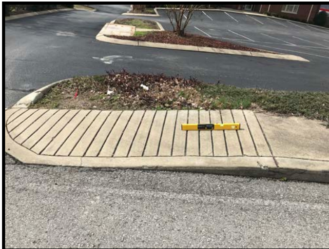
Duke Street- Running Slope of Ramp >8.3\%
