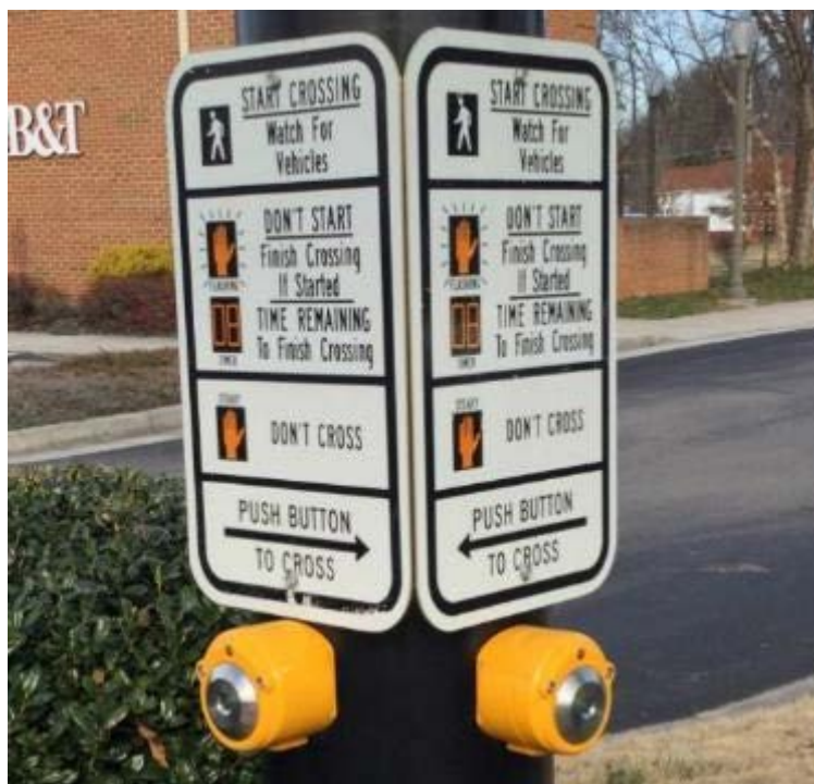
Example of pushbuttons on shared pole
