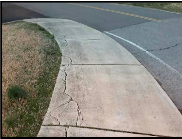
Ruth Street- Cracked Sidewalk and Cross Slope >2\%
