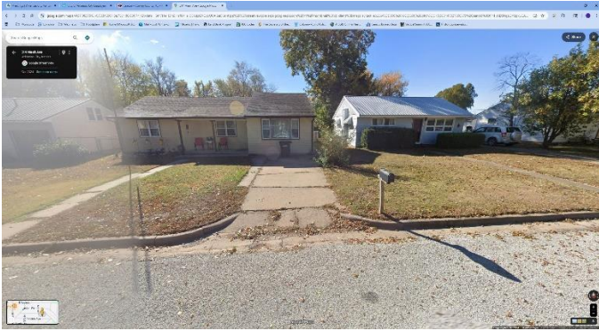
The subject property-Google Streetview October 2024
