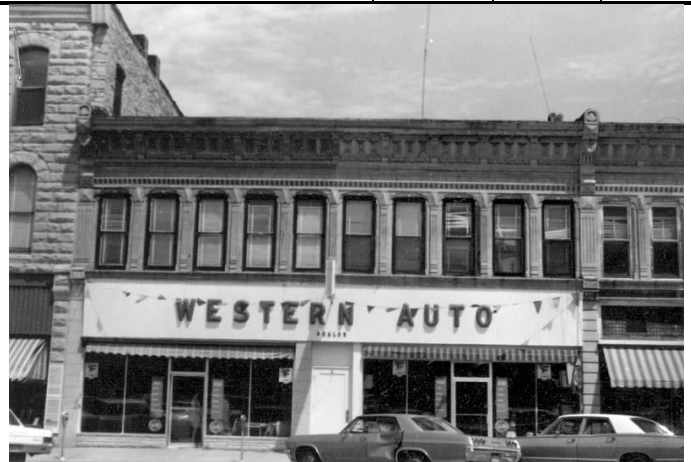
Eagle Block. 312-314 S Summit. Principal Elevation. ca. 1970. Downloaded from KHRI 4/11/22. Existing storefront is in place.
