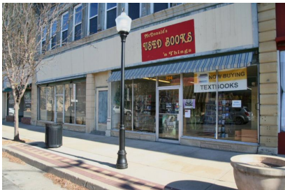
Eagle Block. 312-314 S Summit. South storefront on west facade. 12-11-2017. B. Spencer
