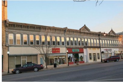
Eagle Block. 312-314 S Summit. East side of 300 block with 312-314 at North end (L). 12-11-2017. B. Spencer
