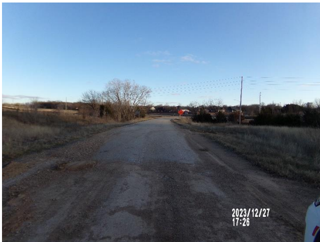
End of pavement approximately 400 feet north of intersection, south of site taken 12/27/2023 by Josh White
