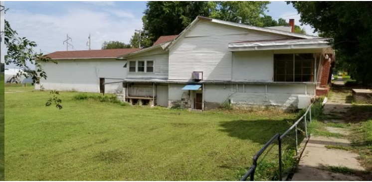
North side of property
