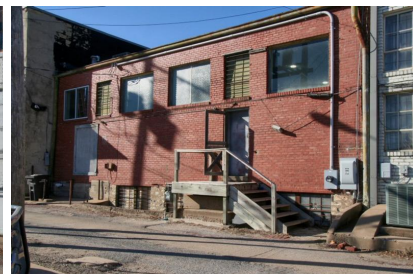
Zadie Building. 206-208-210 S Summit. East/rear facade of 208-210. 12-12-2017. B. Spencer
