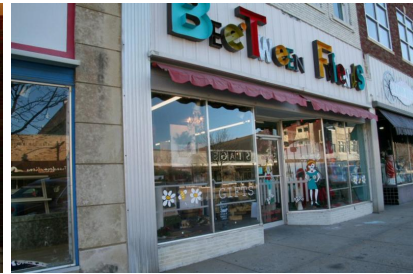
Zadie Building. 206-208-210 S Summit. 206 storefront on west facade. 12-12-2017. B. Spencer
