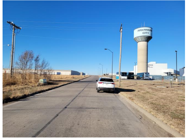
Looking to the west along Goff Industrial Park Rd
