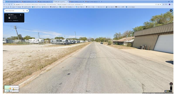
Looking North along 8 th Street. Subject property on the right. Google Streetview from September 2023.
