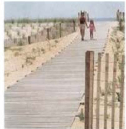
Sand Dune Preservation Modular Walkways.
