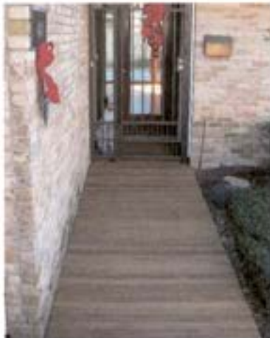
Over Old Concrete
