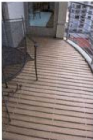
Over a Concrete Balcony
