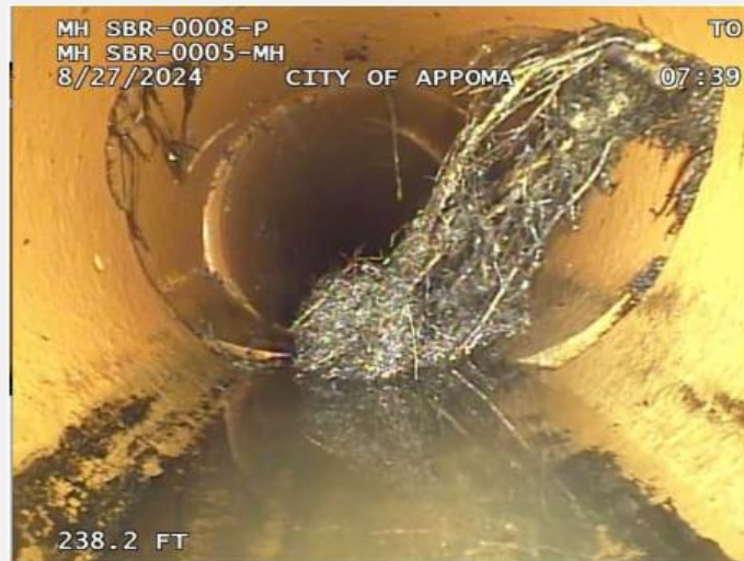
SBR-0006-SBR-0005 – Multiple fractures with roots
