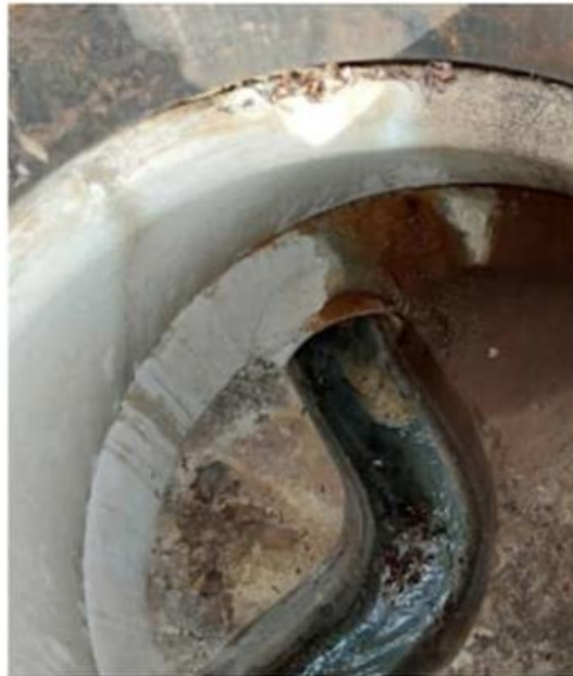
PS5-A-0001-MH: Seal precast joint
