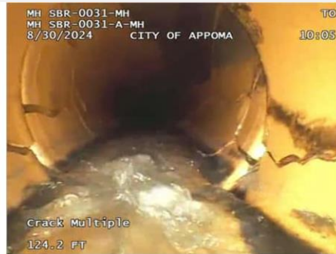
SBR-00031-SBR-0030 – Multiple cracks and fractures
