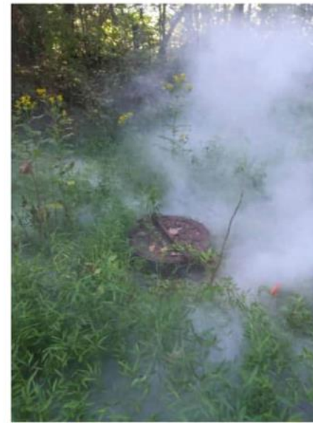
EDA-0014-MH: Unsealed and offset frame
