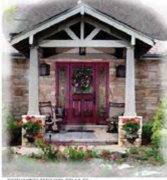
EXPOSED WOOD BEAMS
