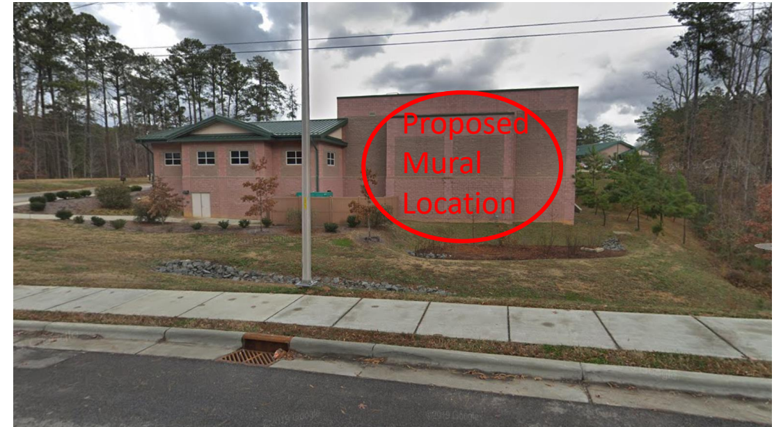
Apex Public Works Building – Route 55
