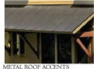
METAL ROOF ACCENTS
