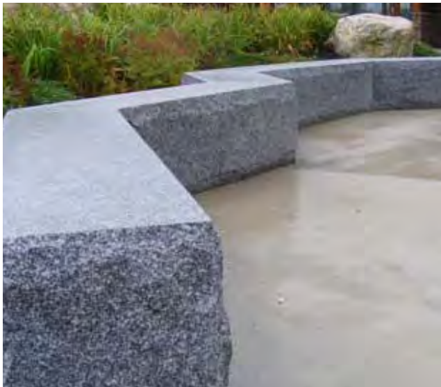
^ Granite seat block with split face sides and smooth top. May include mounted seating.
