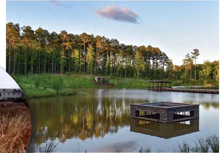
Infrastructure associated with stormwater, such as outfall structures and trash racks, shall be screened with vegetation and/or enhanced with decorative masonry applications.
