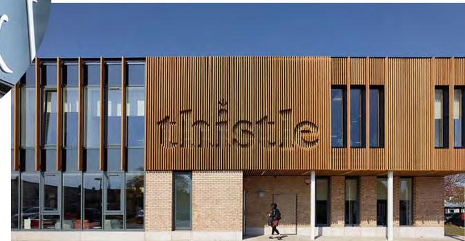
↗ Side mounted to building wall
