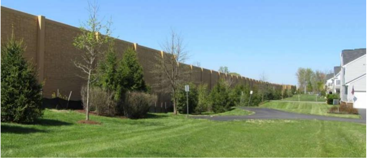
Example of Sound Wall
