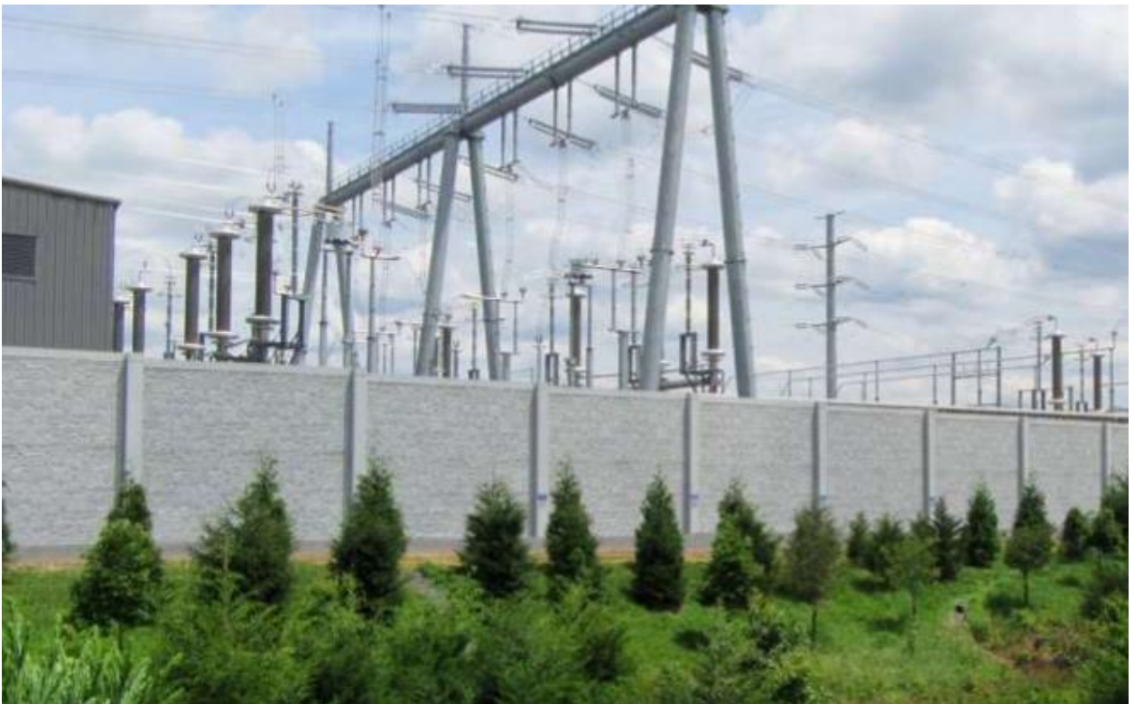
Example of Sound Wall
