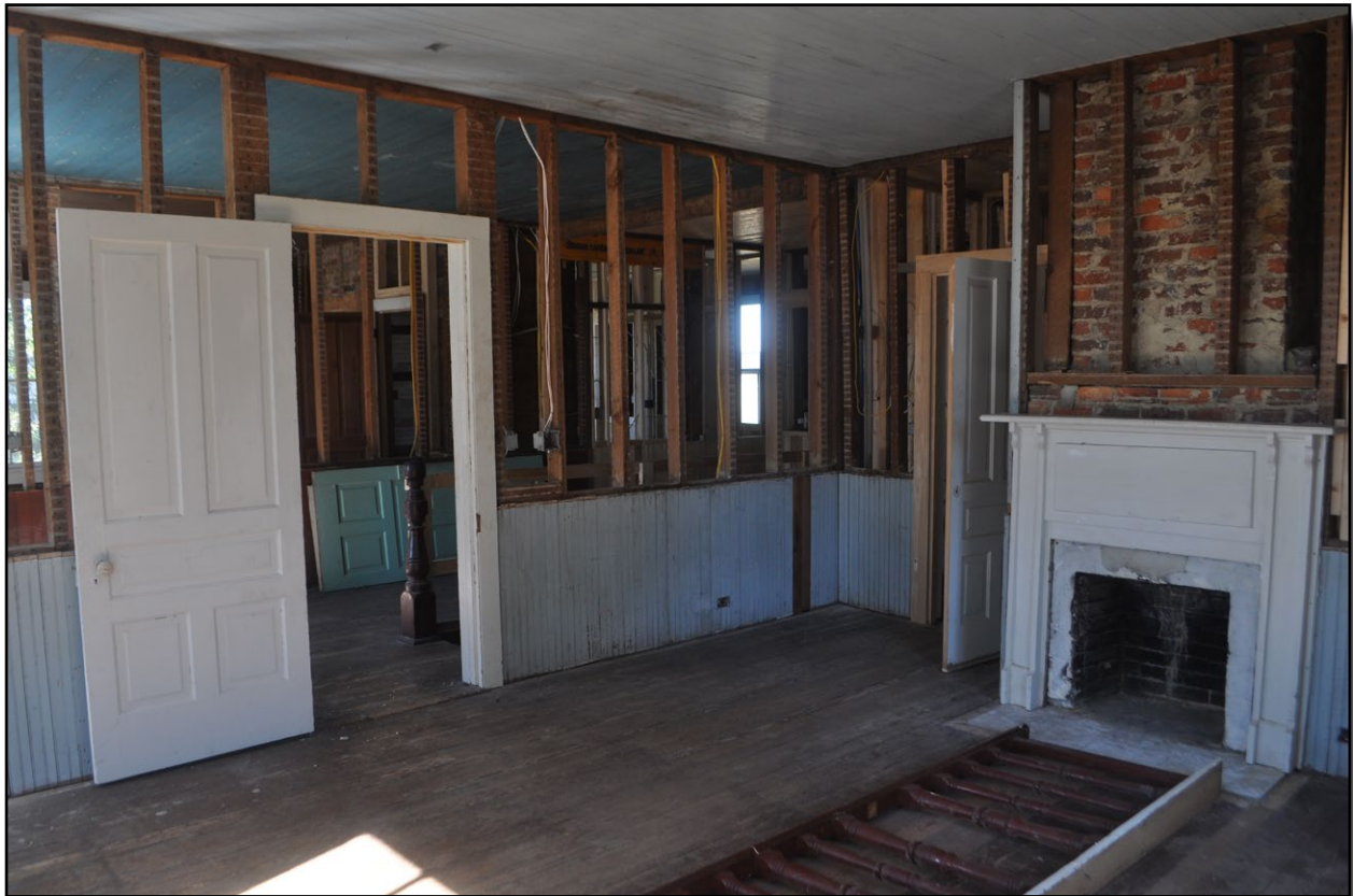
Plate 7.a.9: Second floor bedroom showing mantel, typical 5-panel door and beadboard wainscot.
