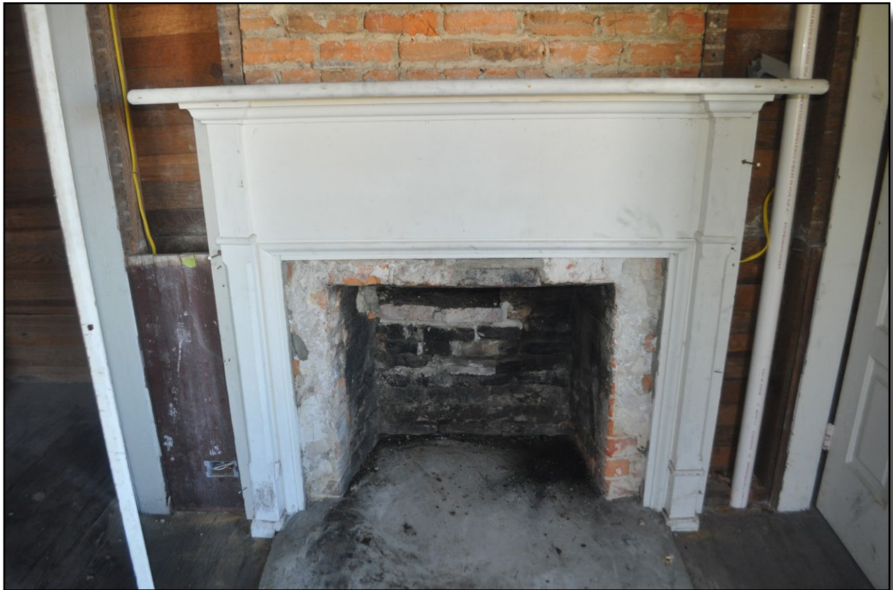
Plate 7.a.8: First floor bedroom fireplace.
