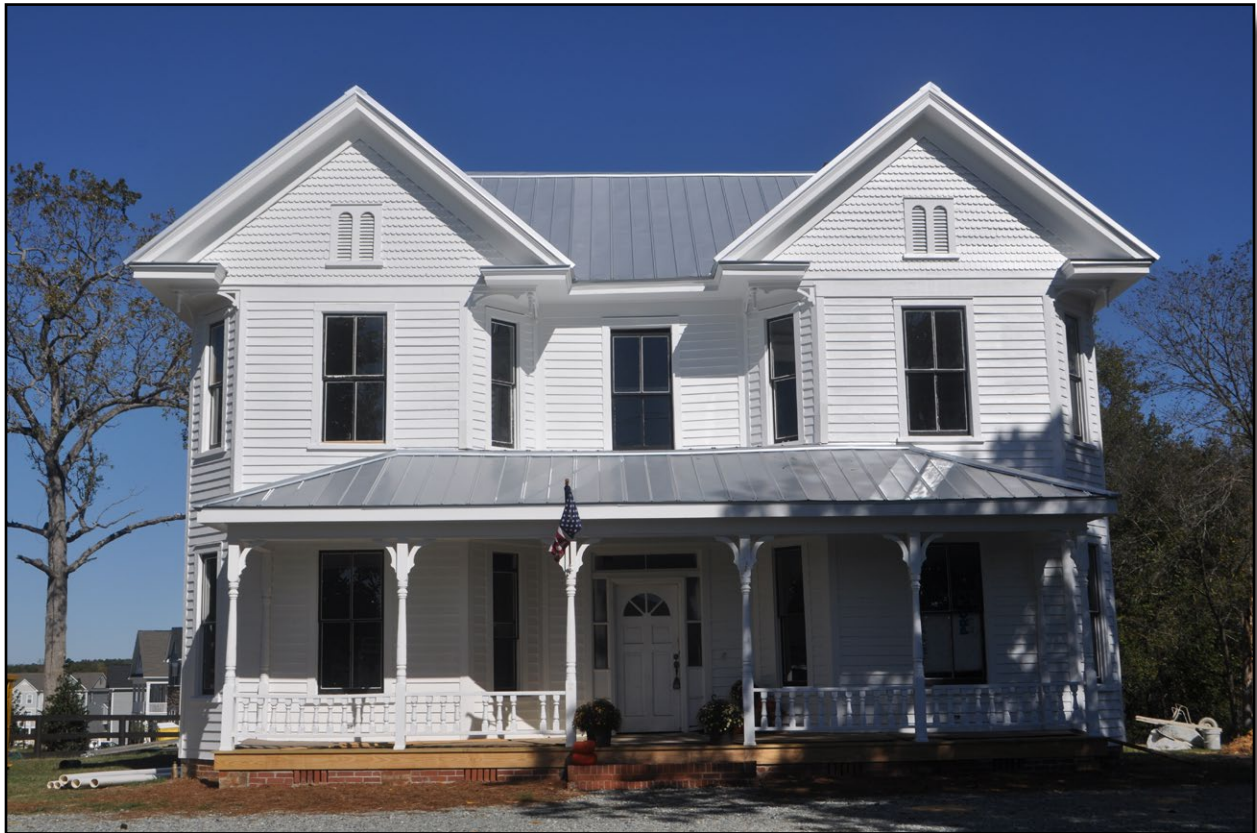
Plate 7.a.1: South elevation, front of the house.
