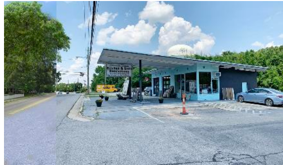
▲ Existing Former gas station building adaptively reused currently as a kitchen and bath renovation business
