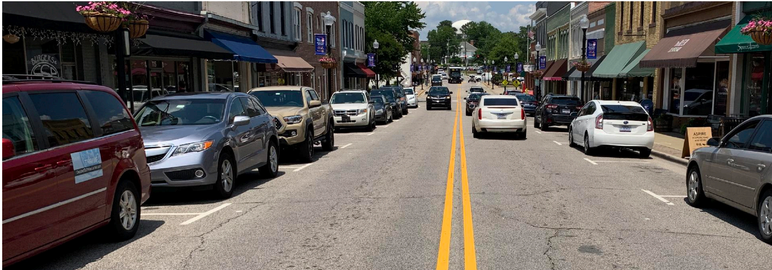
Existing view looking north on Salem Street characterized by narrow sidewalks, no street trees, and relatively tight parking conditions
