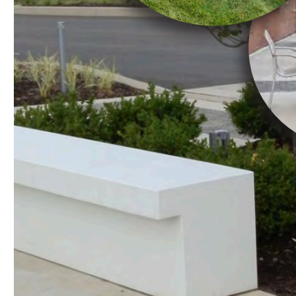
➤ Precast seat walls shall contain lipped edges for comfortable seating. Anti-skateboarding measures may be applied if appropriate.
