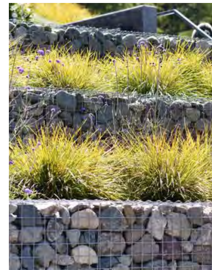
^ Gabion walls shall use large sized, brown and tan toned, smoothed aggregate. Use of gabion walls subject to the approval of the Town of Apex.
