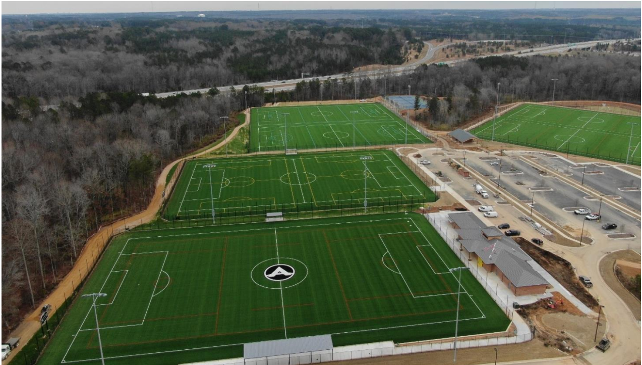
FIGURE 6: SIGNATURE FIELD AND FIELDHOUSE WITH 5 ADDITIONAL MULTI-PURPOSE FIELDS FOR PLEASANT PARK IN THE TOWN OF APEX
