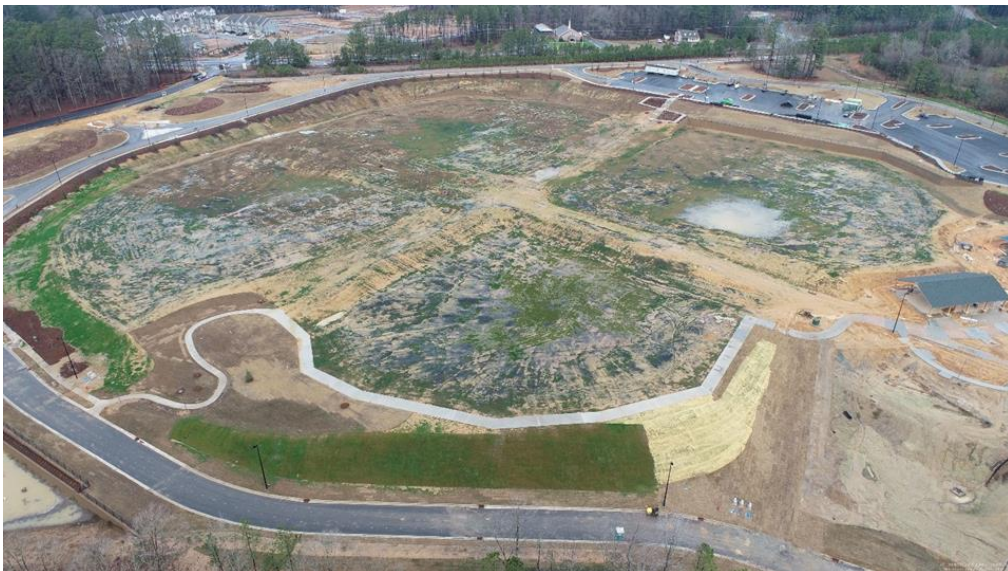
FIGURE 8: AREA OF FUTURE BASEBALL/ SOFTBALL COMPLEX (PHASE 2) FOR PLEASANT PARK IN THE TOWN OF APEX.
