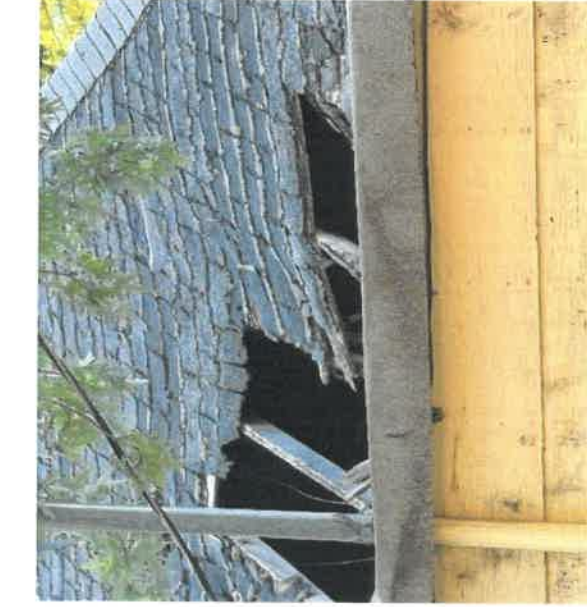
Collapsed and bowing roof due to deterioration-4-903 (e),(f),(g)
