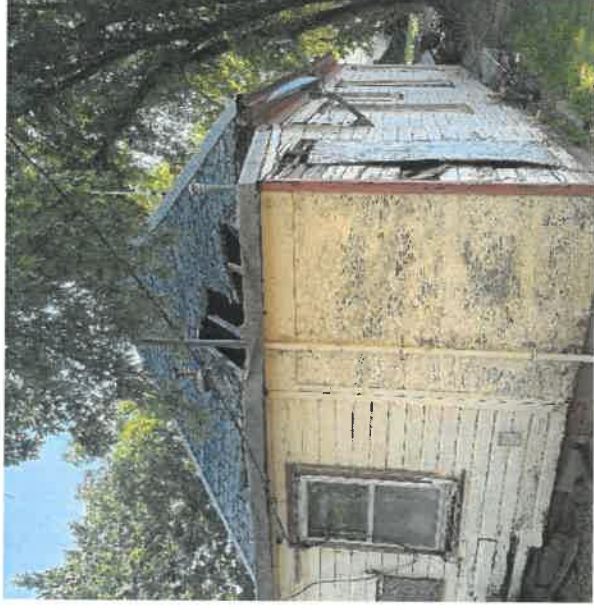
Collapsed and bowing roof due to deterioration-4-903 (e),(f),(g)
