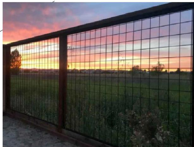
HOG WIRE FENCING WITHIN METAL FRAMED PANELS
