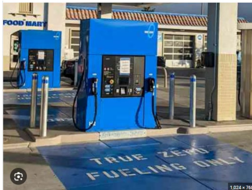
Figure 1: Hydrogen Fueling Station
