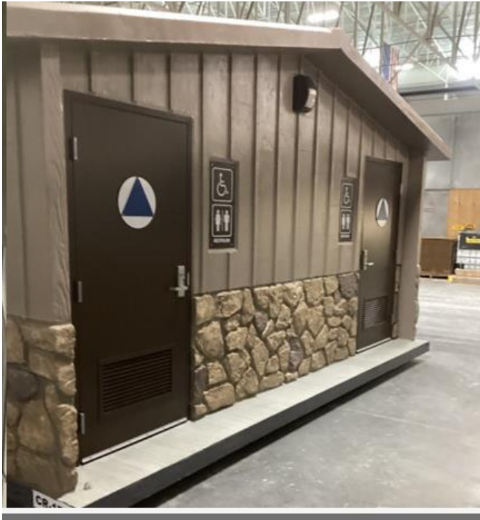
Figure 2: Utica Park New Bathroom (Actual, Constructed)
