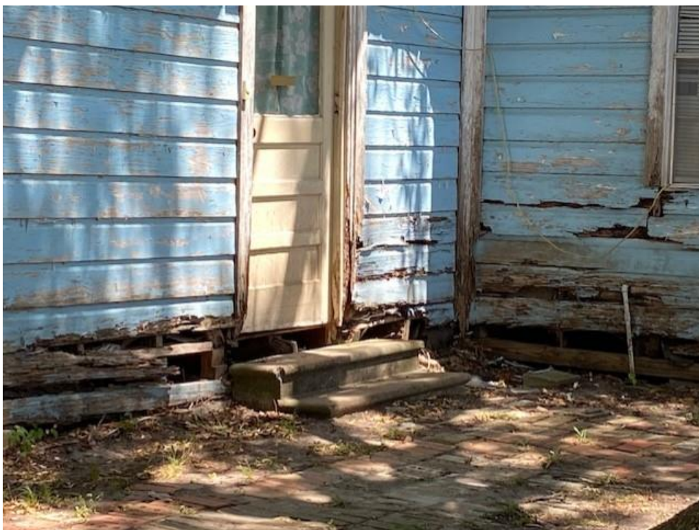
Front close-up – extensive wood rot
