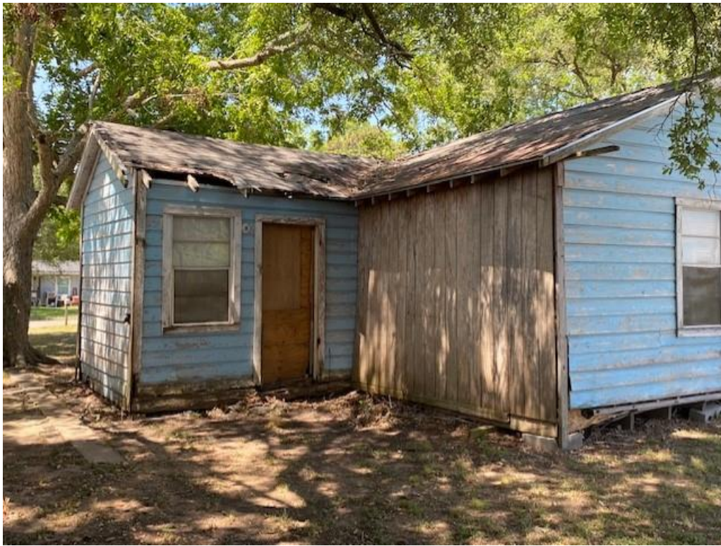
SW corner of structure missing siding, boarded up.
