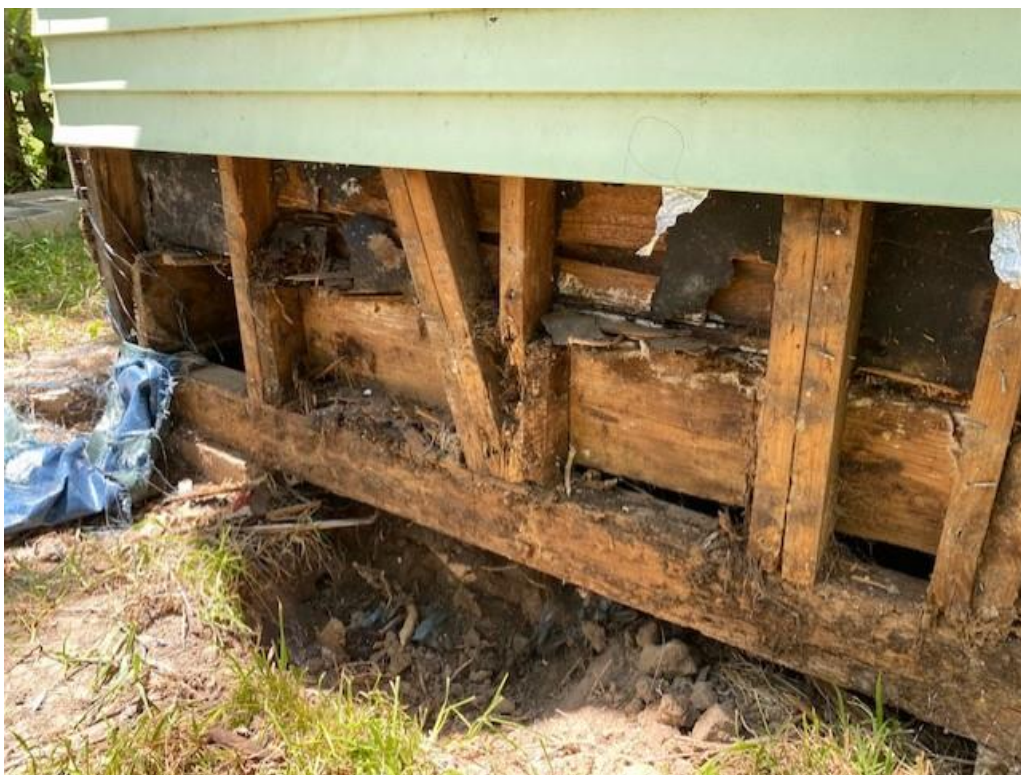
Structural wood rot and missing siding
