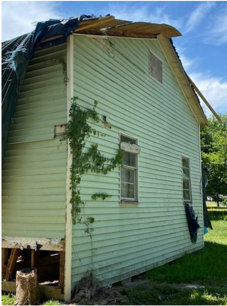
East side of structure - no roof eaves, missing floor, broken windows, missing/rotted siding
