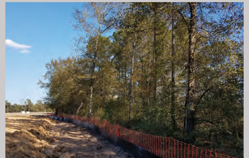
Example of dual-purpose tree preservation by combining silt and tree protection fencing allows for a smaller footprint and aids in reducing construction cost.
