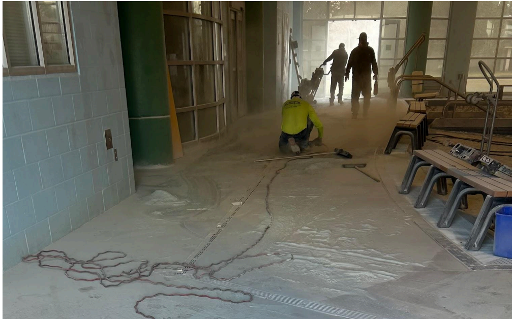
Tile & Deckings: pool decking removal and tile bead blasting started January 19th week.
