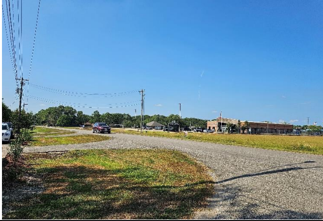
View looking East toward the Subject Site
