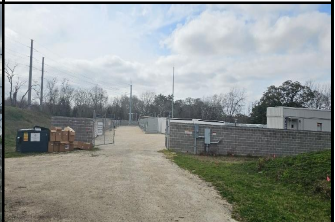
View looking west towards Site Entry
