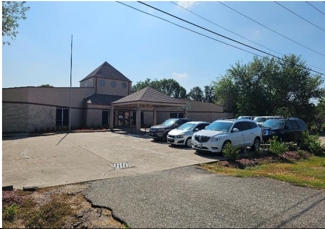
View looking West across from Site (Daycare)
