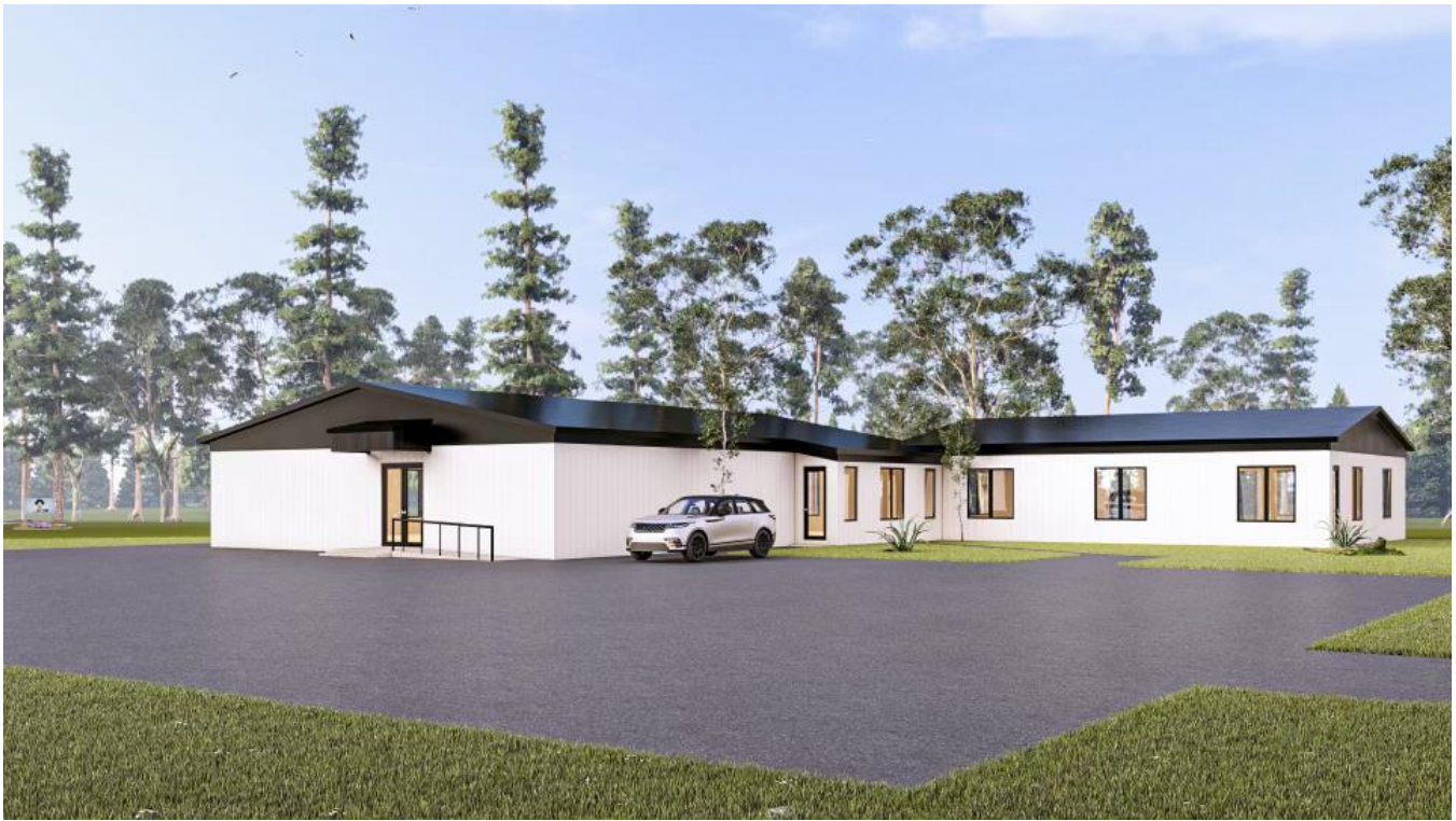
Proposed building side and parking lot
