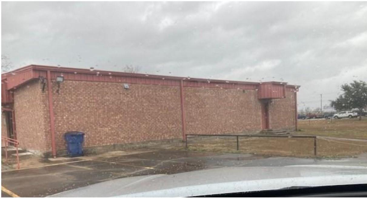
View of building side from parking lot
