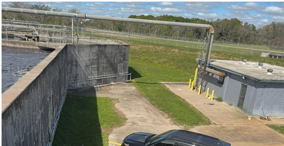
Figure 4 View of the Blower Building from the Southeast
