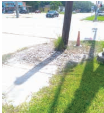
Existing Cracked Sidewalk and Poor ADA Facilities
