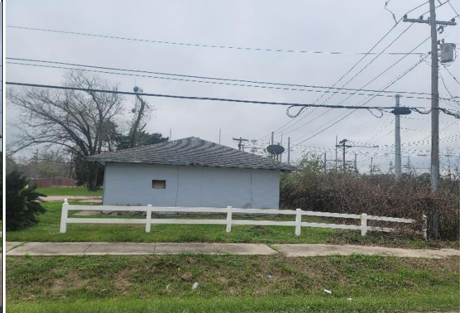
VIEW LOOKING SOUTH AT PROJECT SITE
