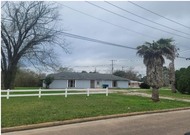
VIEW LOOKING WEST AT PROJECT SITE
