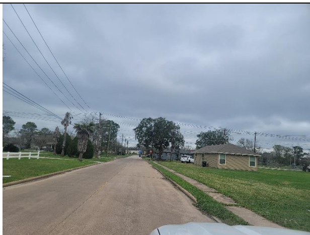
VIEW LOOKING NORTH ON WALKER ST.
