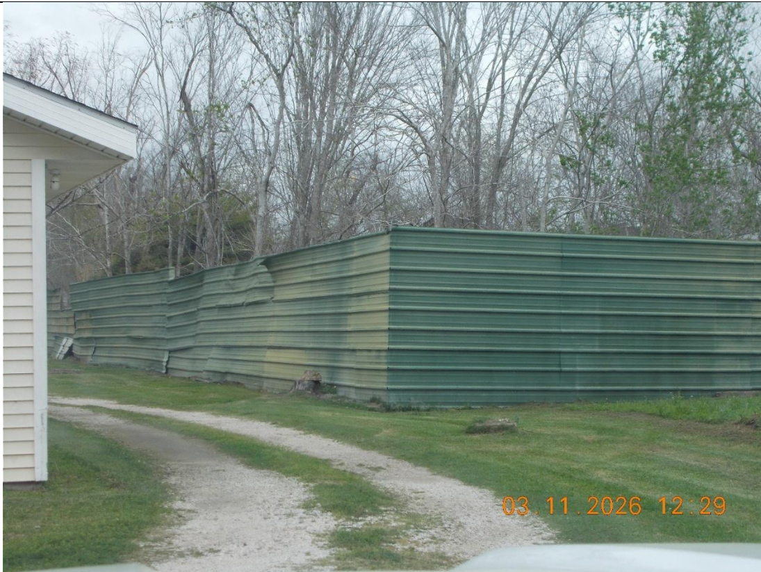
View looking along driveway toward rear and neighboring fence
